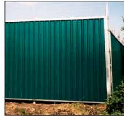
"Big Brother" used standard 2.4m High Steelhoard, with additional Barbed wire toppings, as well as a non standard 3m High system.
