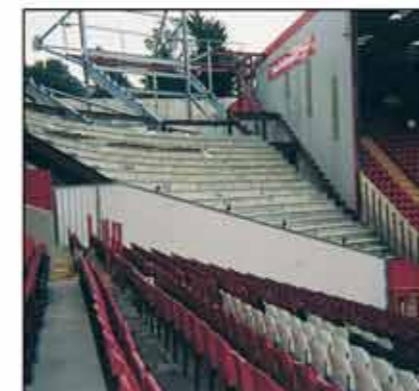
Crowd loaded Steelhoard has been developed to protect the public at a number of football grounds and is calculated to withstand 5kn per metre.
